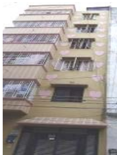
Fig. 4. Smaller unit size building at Mirpur area
